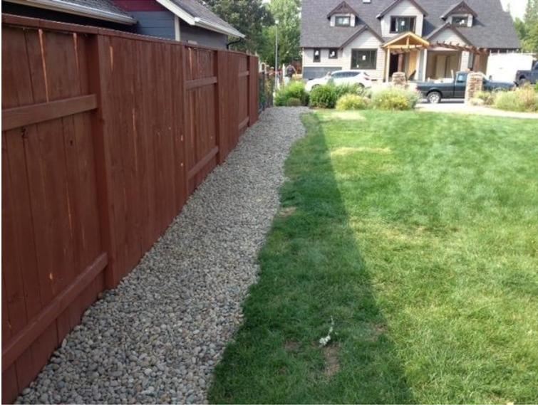
At Ponderosa Park, Public Works constructed an underdrain system. The park has experienced ponding of water from irrigation and during the winter. The new drainage system will prevent any damage and enhance the park.
