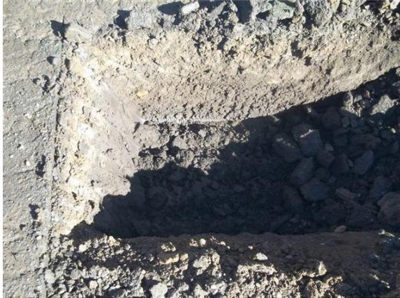
A minimal amount of asphalt was discovered over the existing clay. To preserve the pavement and alley, a full structural section of asphalt,  $\frac{3}{4}$ " and 4" rock was recommended by the engineer. It was hoped the section could have been reduced by discovering better suitable soil. The project is scheduled to advertise mid February.
