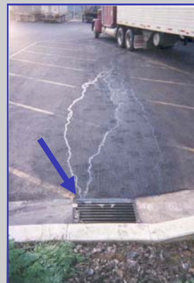
Oil from parking lot entering storm system
