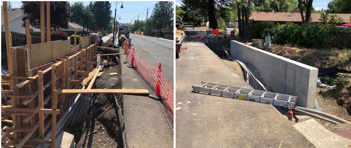
Headwalls were poured over the Buchanan channel.
