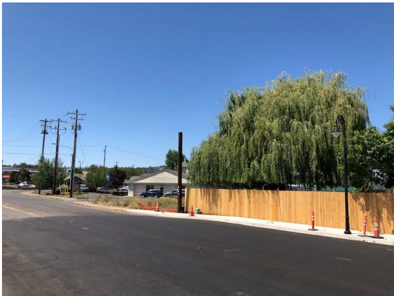
Hunter Communications removed their last overhead line.
