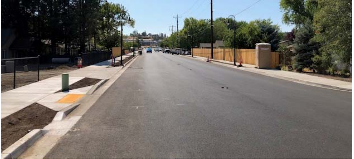
Central Pipeline poured additional sidewalks, driveways and ADA ramps.
