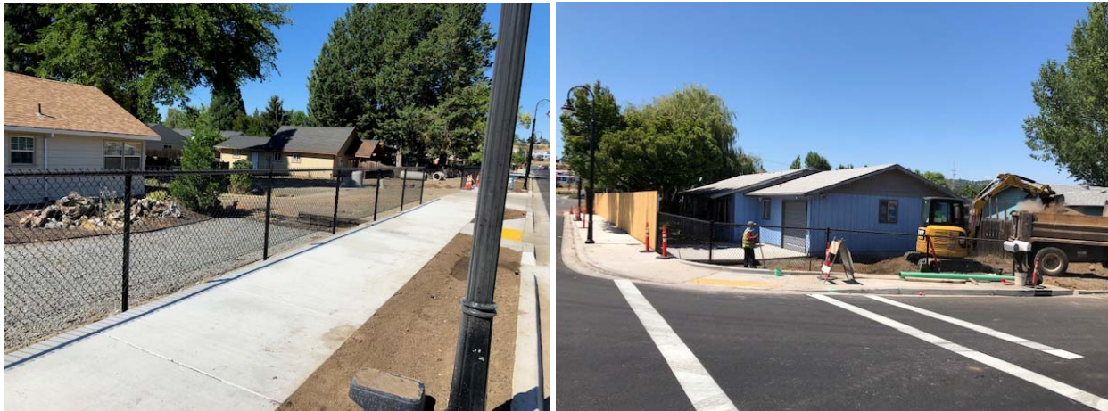
Quality Fence continued placing fencing throughout the project.
