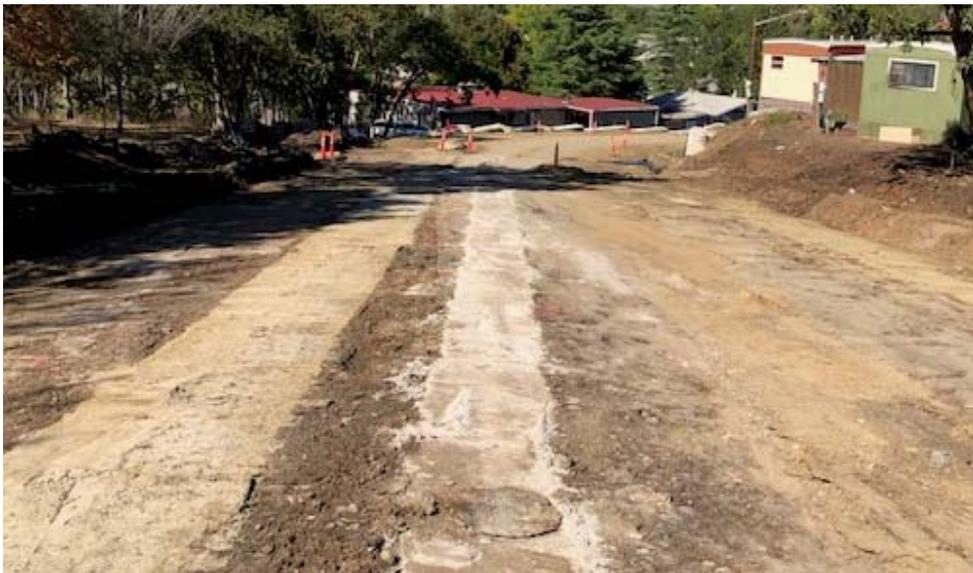
The road bed is prepared for placement of base and subsequent paving.
