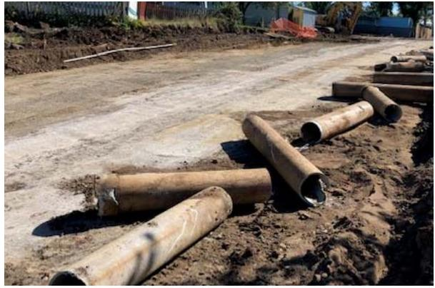
The existing storm up the hill was removed for the road widening.
