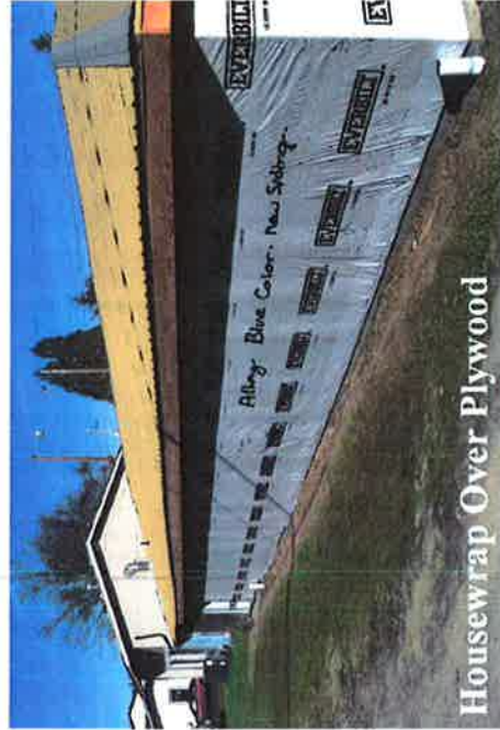
New Plywood Sheathing and Roof
