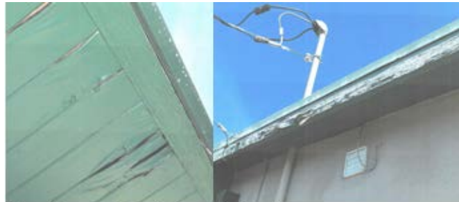
Deteriorated fascia boards & paint
