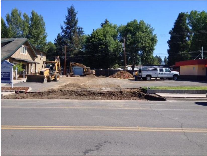
The existing driveway was removed to place a commercial driveway. The driveway is thicker to accommodate delivery trucks, and wider to allow multiple vehicles to use the driveway. Previously only one full sized truck could use the driveway to enter the Judge Stewart House and Main Event parking lot. Installation of the storm system and paving will complete the project.
