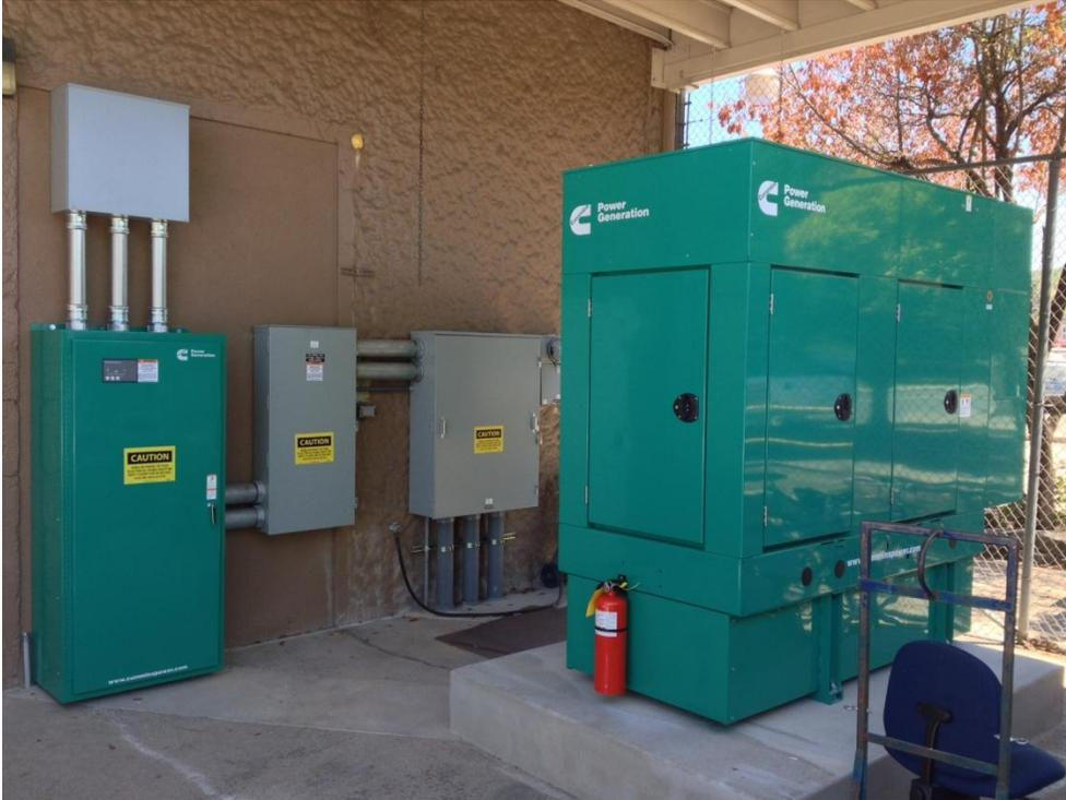
The portable diesel generator was configured to provide backup power to the Bellerive Pump Station, in the event of a power outage.
