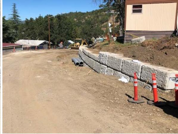
The Ultrablock retaining walls were completed for Stage 1.
