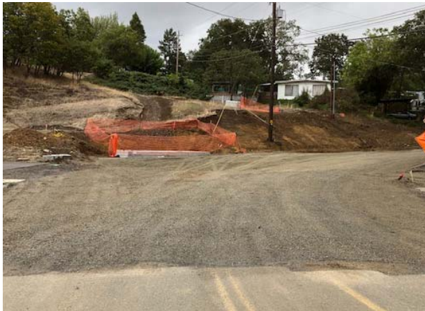
Excavation and placement of the new base for E. Main Street/Stevens Road.
