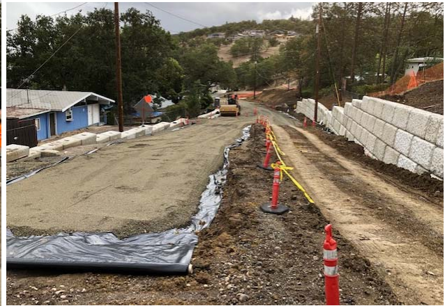
Excavation and placement of the new base for E. Main Street/Stevens Road.
